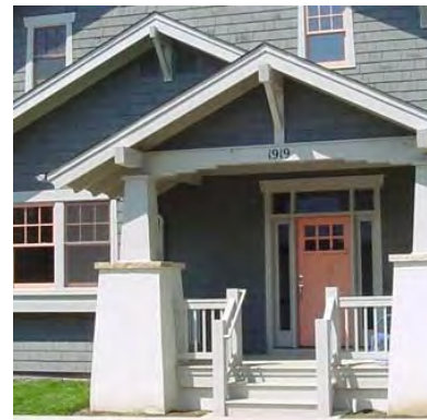
Detailing is appropriate to style of architecture.
