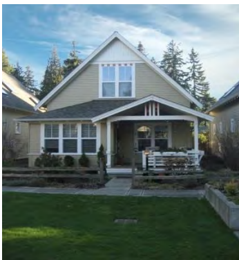
Entries including door, windows and porch, should be given special attention.
